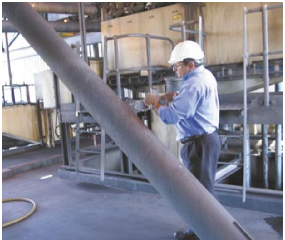
Hard water such as the process water used in North Goonyella coal treatment plant causes scaling on galvanized coatings, which have still retained their original thickness (over 100 microns) after 12 years of operation.
